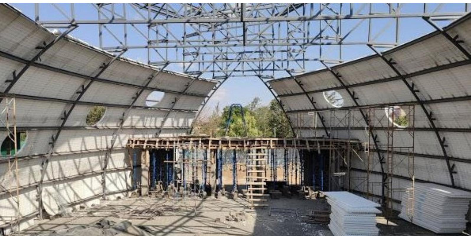
Fig 11: The interior volume of the church enclosed by steel and EPS to give maximum volume.
