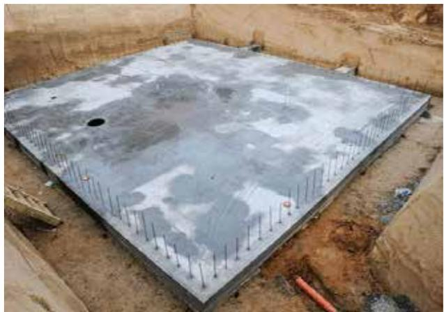
A slab foundation is a popular choice when the ground is soft and requires an equal weight distribution. However, it is more time-consuming and more expensive to build than a pier foundation.
