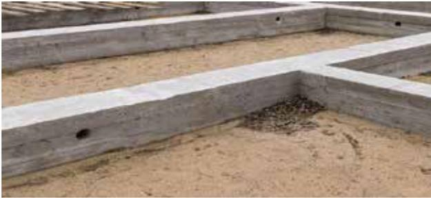
A strip foundation (also known as a trench foundation) is somewhat of a combination of the previously mentioned pier and slab foundation. The strip foundation, shown here, is simply a strip of concrete which is laid to support the containers. The concrete strip is normally 300-600mm wide and 1200mm deep.
