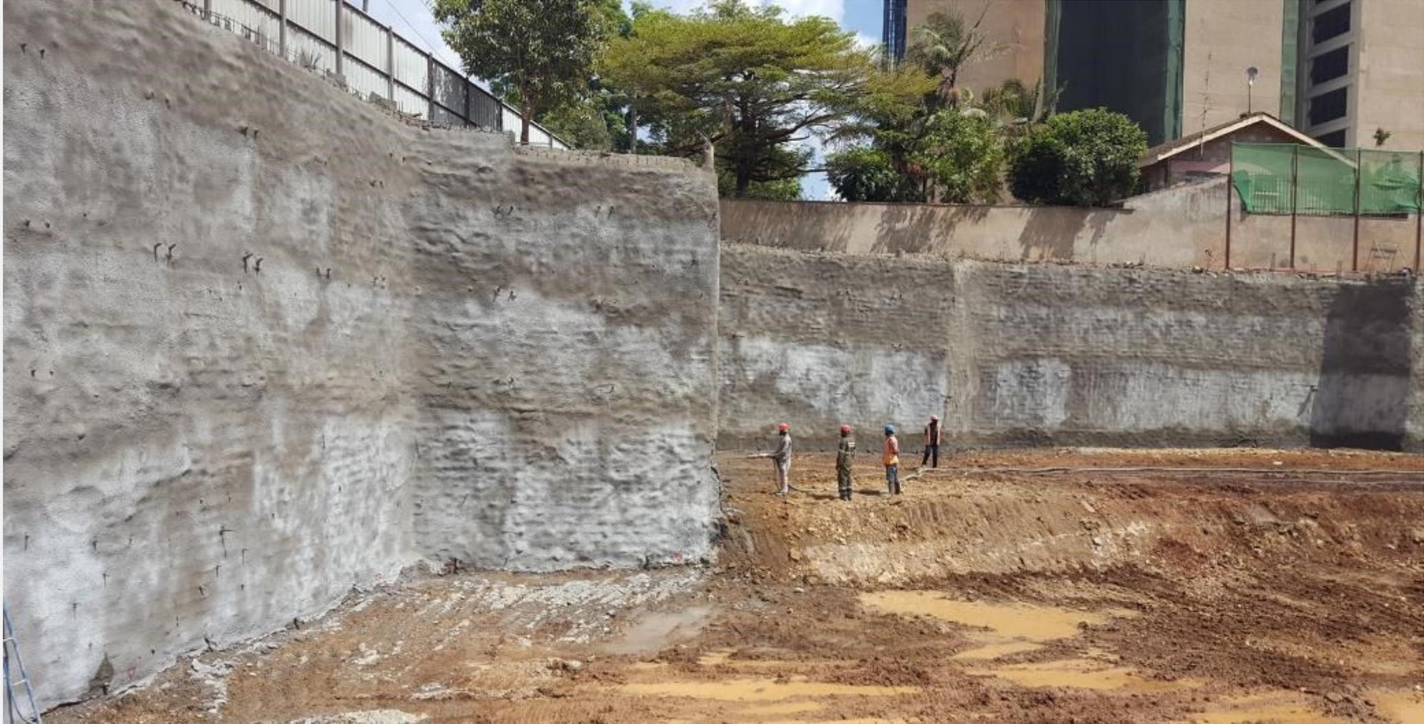
Soldier piles and reinforced shotcrete permanent retaining wall. Note the battered slopes
