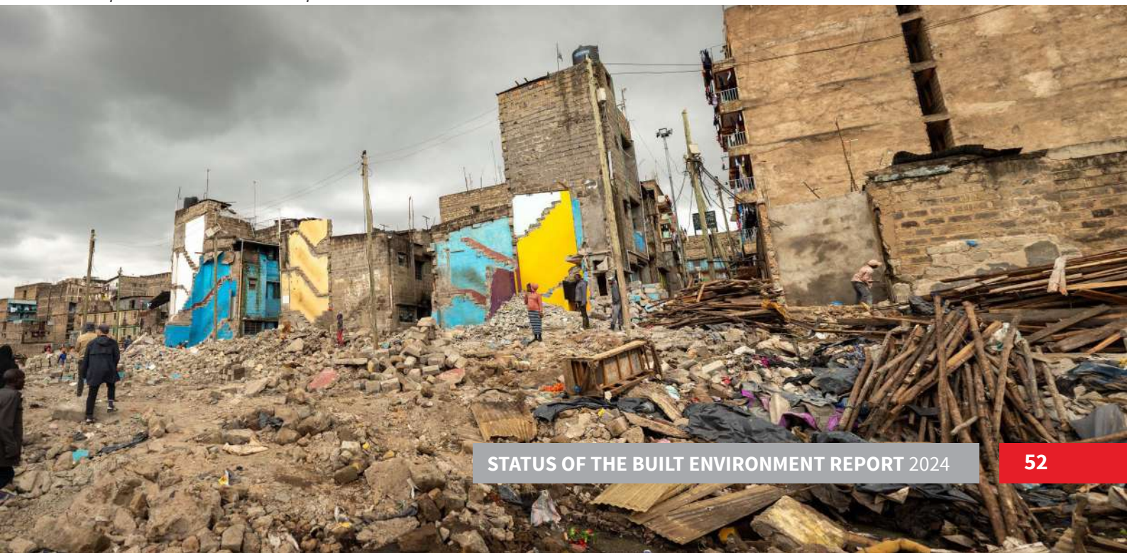
Riparian Demolitions in April
