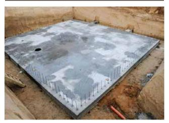
A slab foundation is a popular choice when the ground is soft and requires an equal weight distribution. However, it is more timeconsuming and more expensive to build than a pier foundation.
