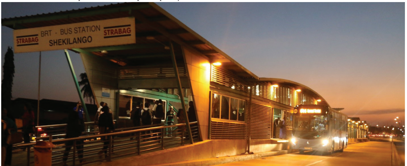
Shekilango bus Terminus along Dar Es Salaam's BRT
