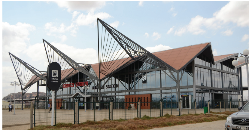
Kibwezi Railway Station, Kibwezi
