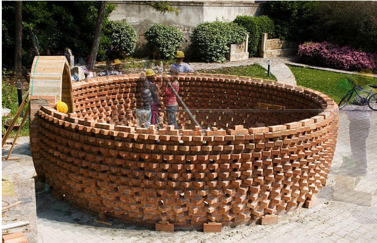
Locally sourced brick
