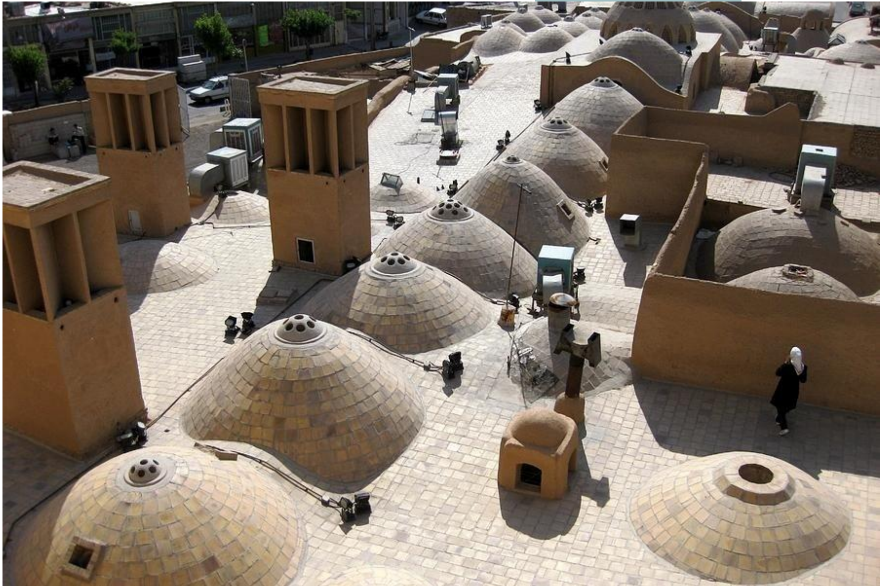
Traditional Wind chimneys (wind catcher/ wind scoop) in Yazd, Iran
