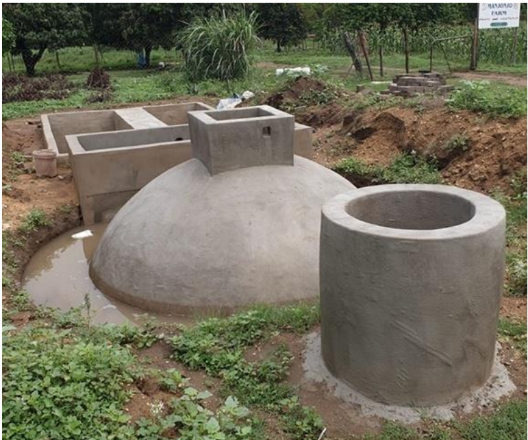
Construction of a Bio-digester plant
