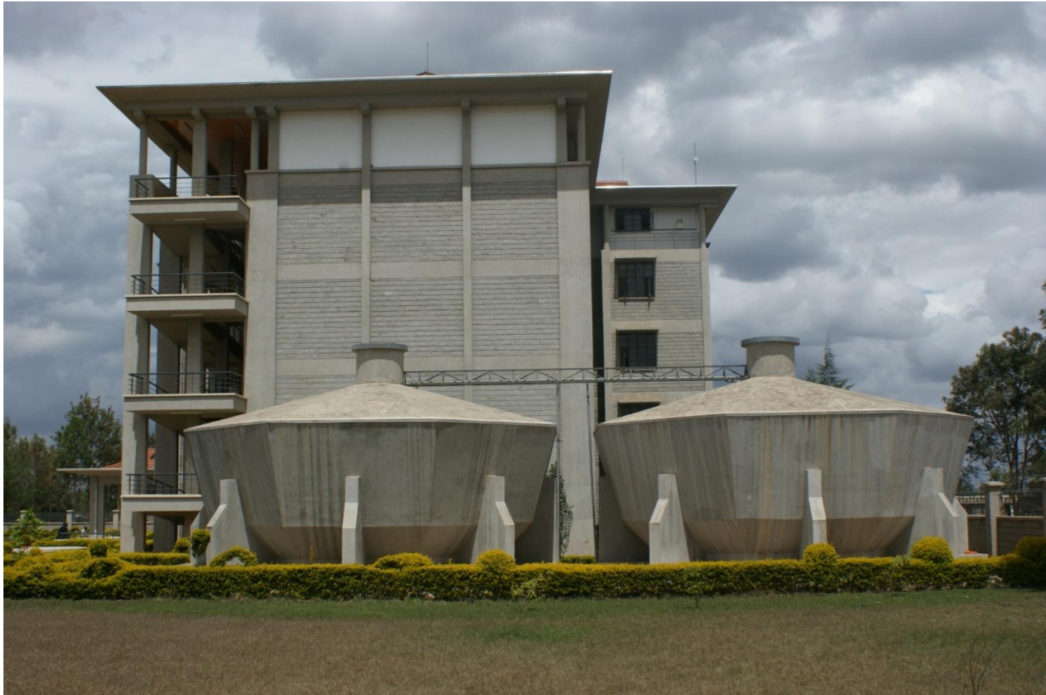
Water tanks next to a building
