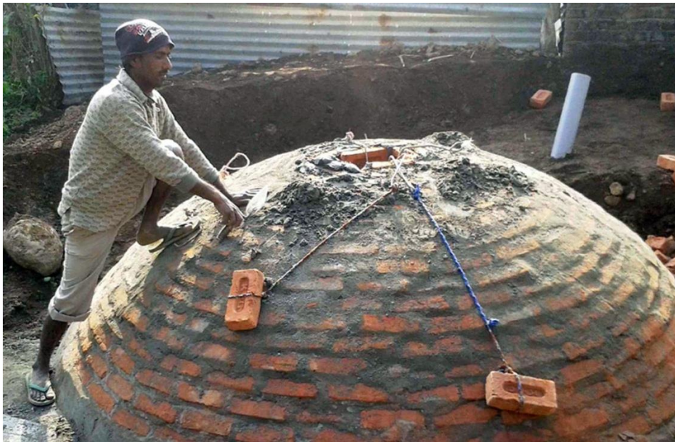
Construction of a Bio-digester plant
