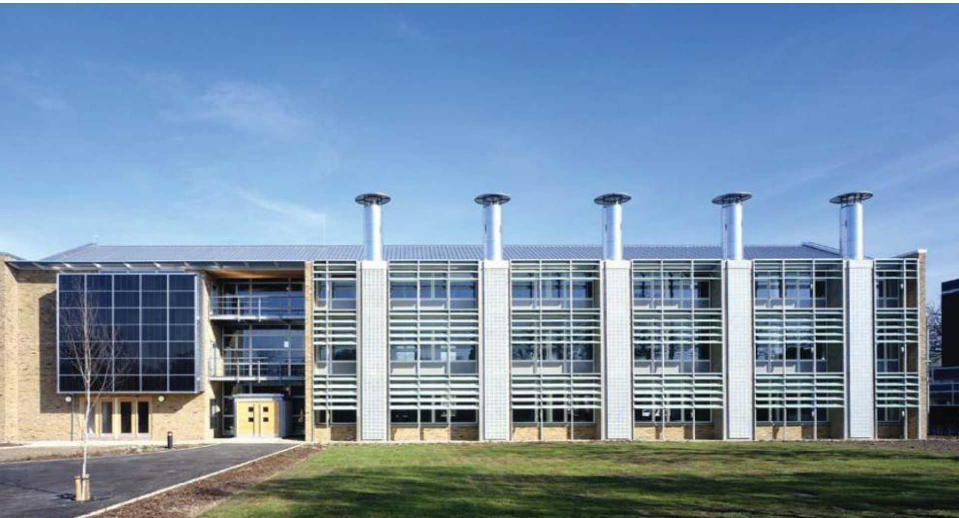
Modern thermal chimneys BRE HEADQUARTERS, Watford London Architects: FEILDEN CLEG
