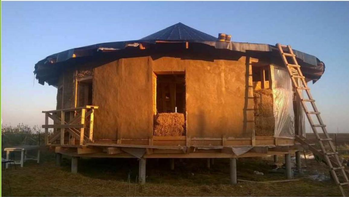
Krasnodar region Timber frame and hay house. Clay stucco.
