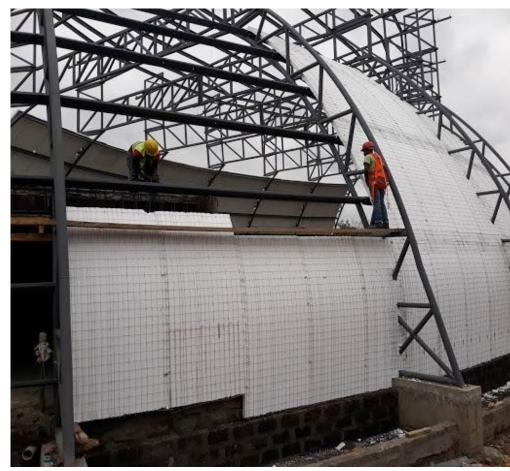
Fig 09: Fixing of the EPS panels onto the curved steel frame supports.
