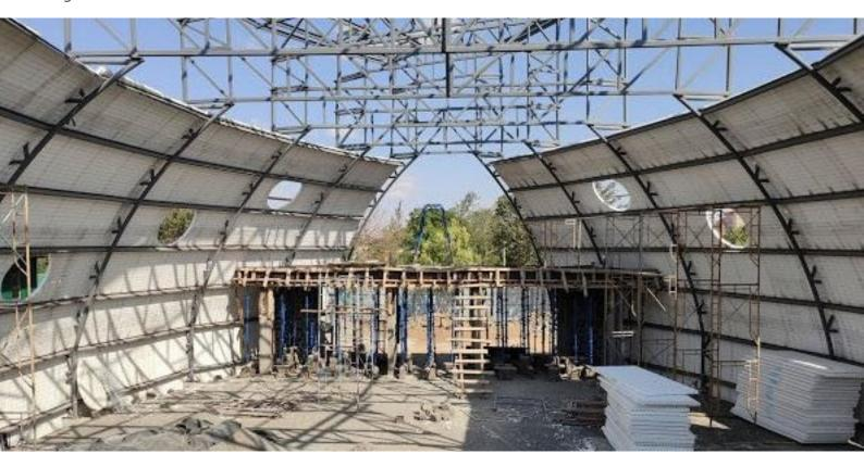
Fig 11: The interior volume of the church enclosed by steel and EPS to give maximum volume.
