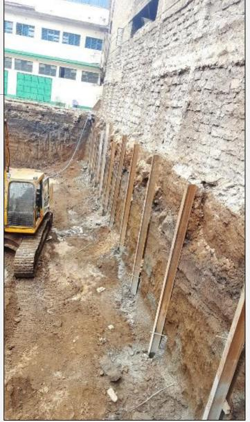
I-Beam soldier piles anchored with sanchors
