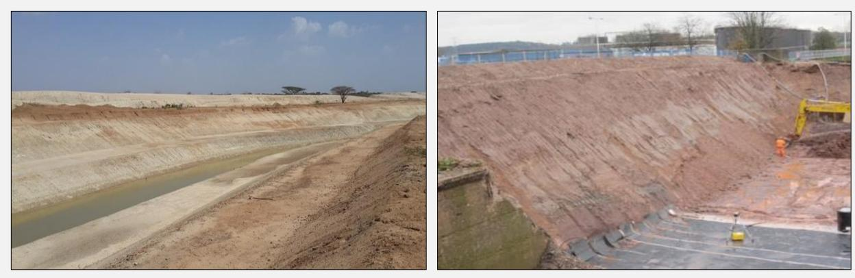
Battered sides of excavated deep trenches & basements
