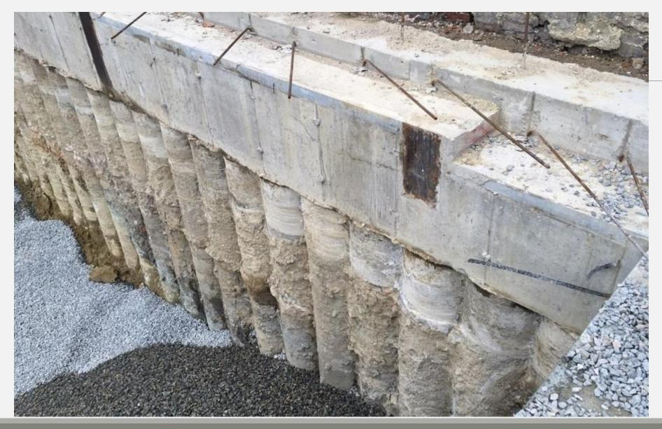
Secant piles with a capping beam
