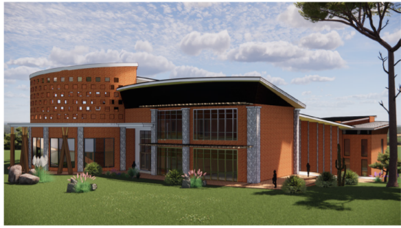
View of the auditorium which takes advantage of the site terrain. Raking follows the contours down the slope.
