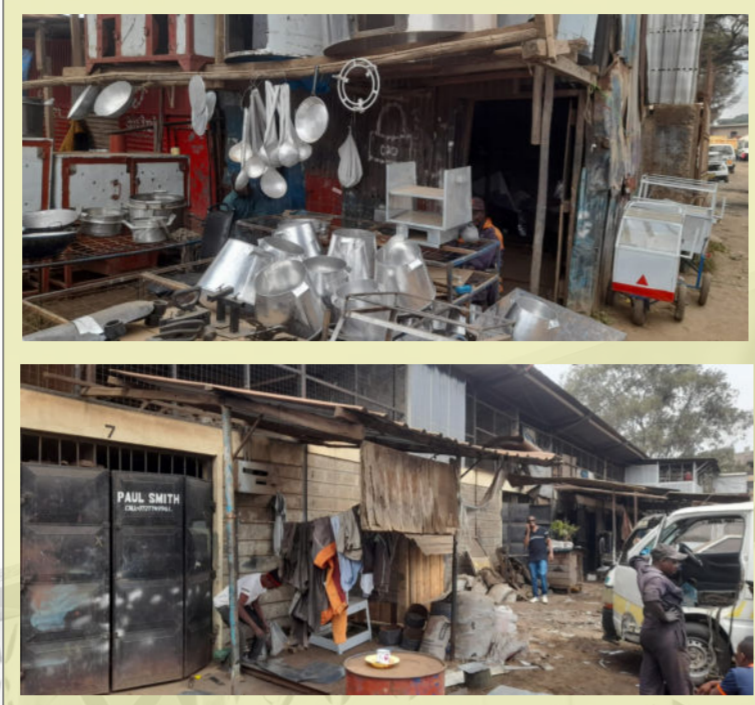
Images showing the various problems in Kigandaini metal works workshops. source- Maria Gicheha 2025
