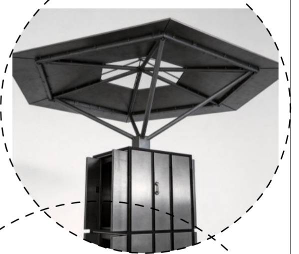
- USE OF STEEL MODULAR RE-POPULABLE UNITS DUE TO AVAILABILITY OF TECHNICAL KNOWLEDGE, ITS LIGHTWEIGHT AND EASE OF JOINERY AND DECONSTRUCTION PROPERTIES
