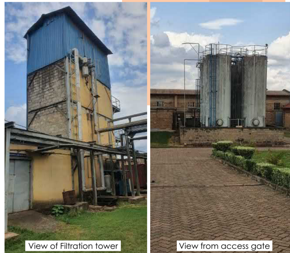
View of Storage tanks
