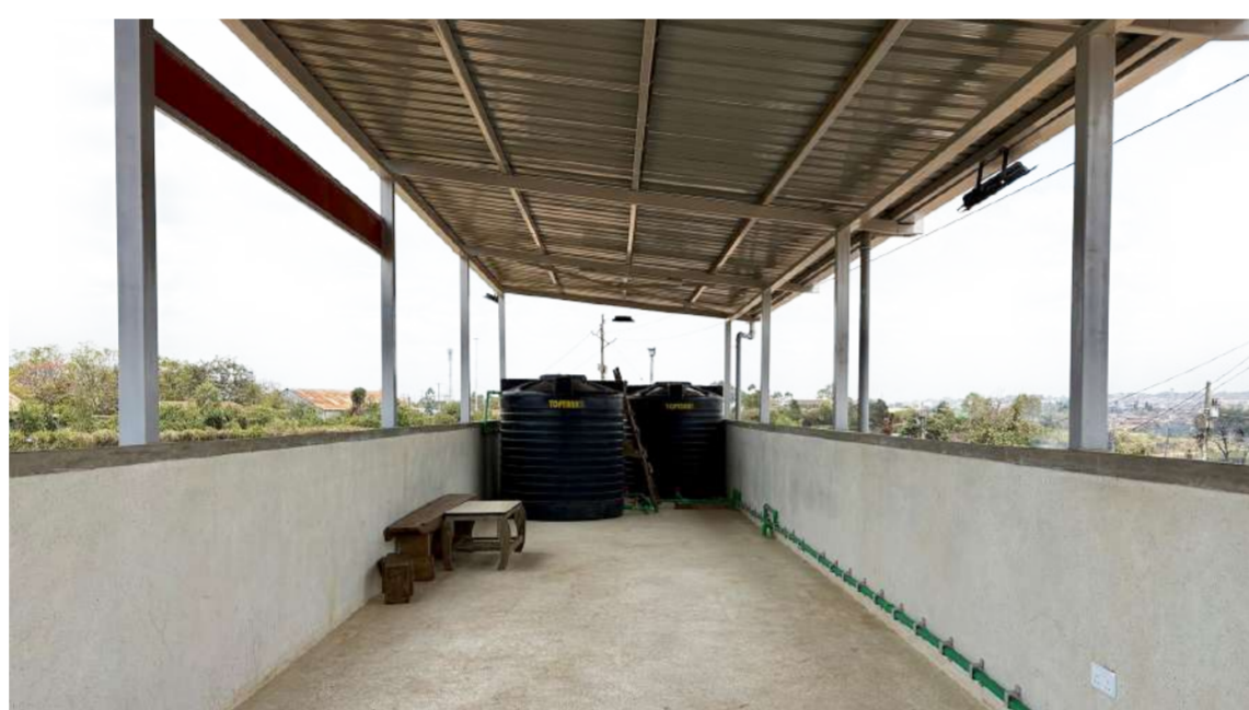
Kaa Soba - Rooftop tank storage
