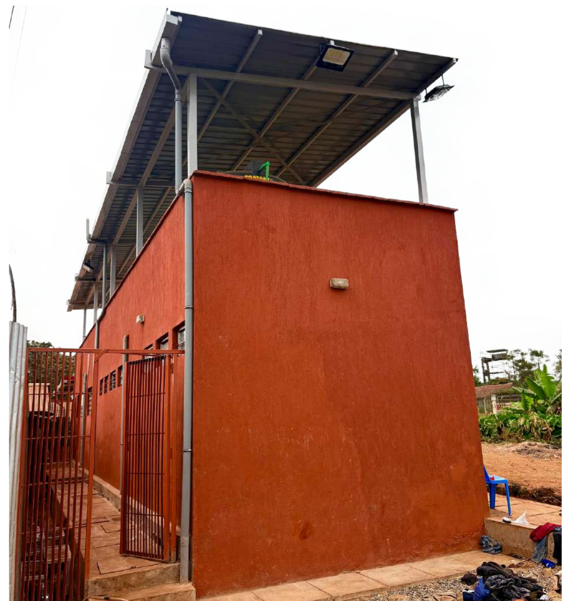
Kaa Soba - Solar security lighting
